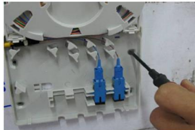
Pic20: fixing the box
